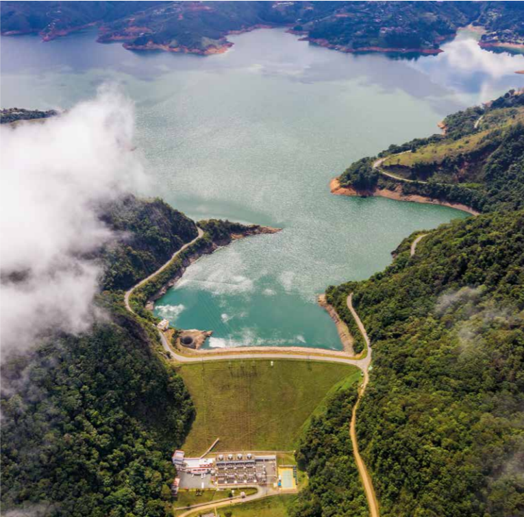
▶ Calima Hydroelectric Plant Valle del Cauca
