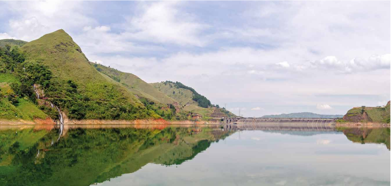
▶ Salvajina Hydroelectric Plant Cauca
